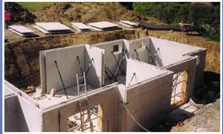
Pre-cast/insitu hybrid walls
