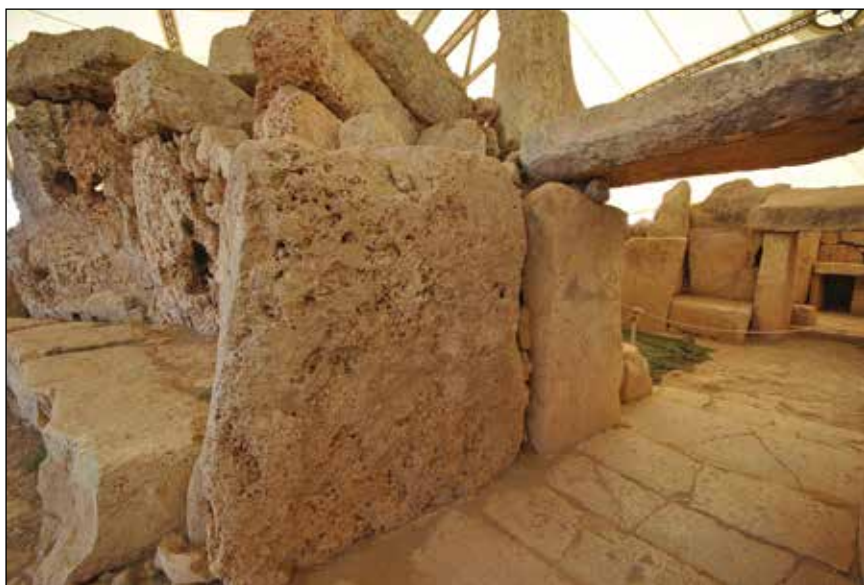
Fig. 6.5: Visible signs of a constructional split in both the threshold and the wall panelling about 2/3 inside the main entrance of the south temple. (Photo T. Lomsdalen).
