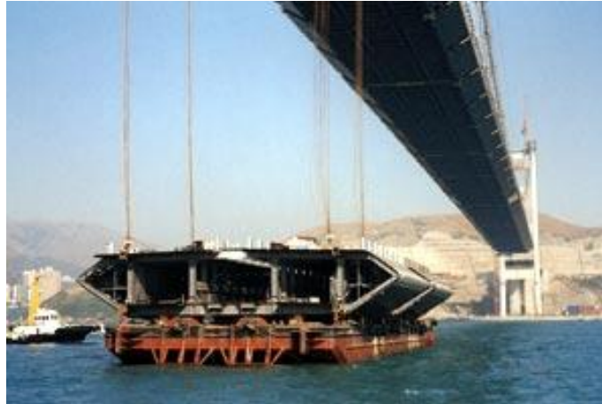
Deck segments being transported under the bridge on sea
