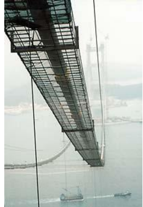
The catwalk suspended on the main cable
