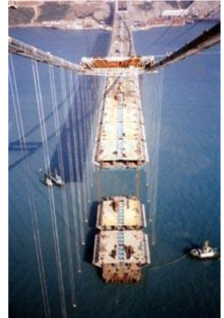
Deck segments being lifted into positions
