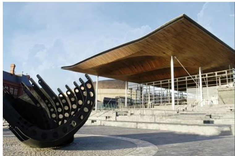
Figure 1- This image shows the exterior of the Senedd Building located in Cardiff Bay. https://senedd.wales/visit/our-estate/the-senedd-a-landmark-building/
