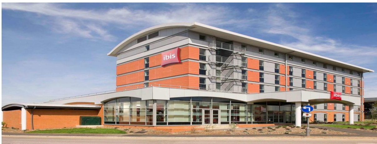
Figure: IBIS Hotel – Borehamwood (2025)
