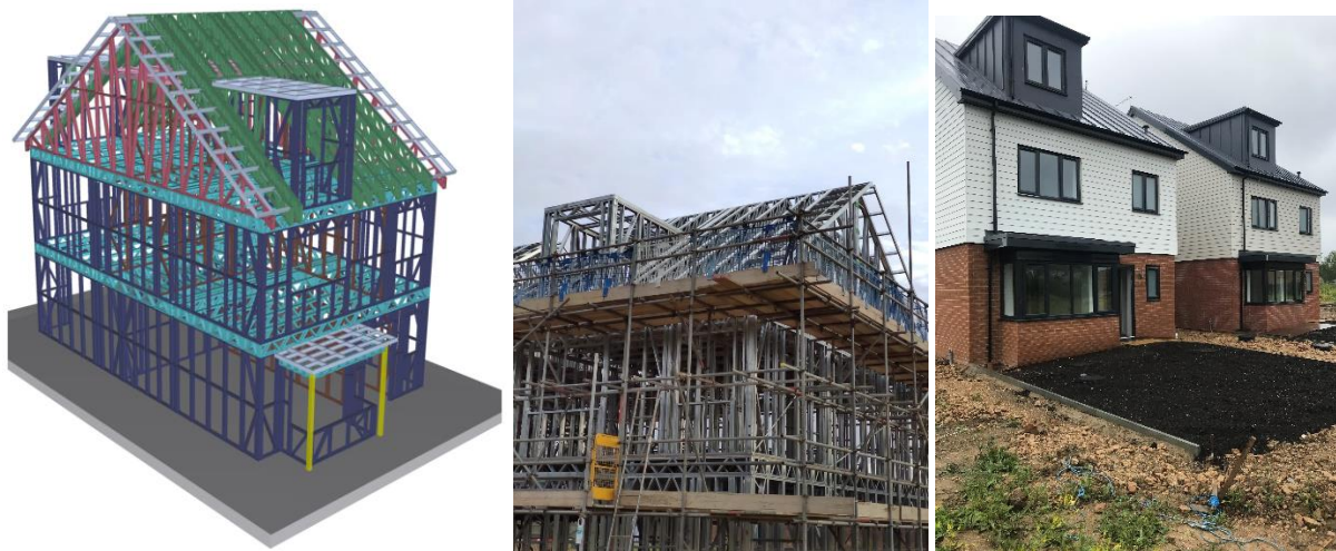
Osprey Developments, March, Cambridgeshire - Industry 4.0 aids customisation of housebuilding.
