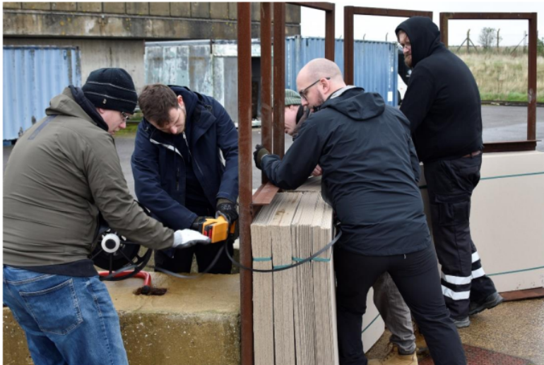
Figure 10: Strawboards being put in place.
