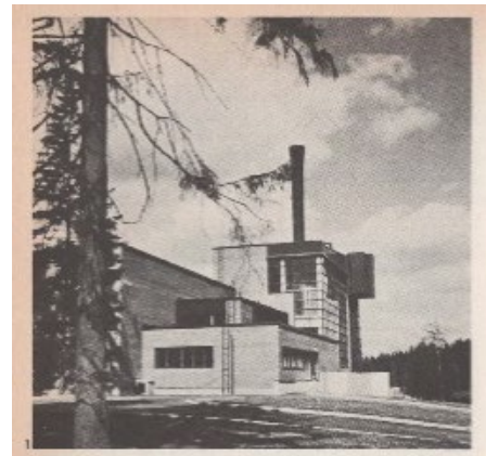
Figure 16: Otaniemi Heating plant perspective view (Aalto, 1975 pp. 146-147)
