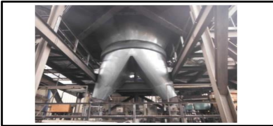
Figure 4 - Cyclone Discharge Legs (Trouser Legs)
