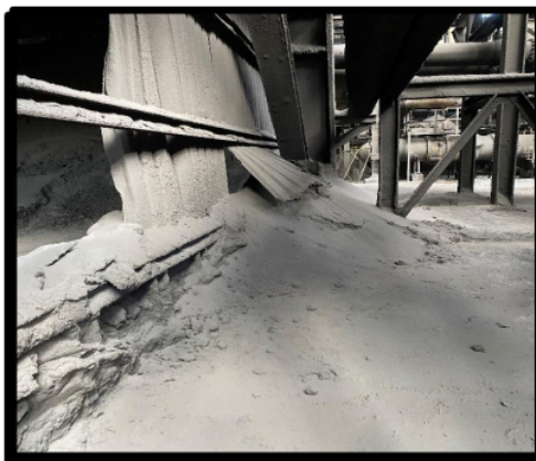
Figure 7 - Pug Mill Floor
