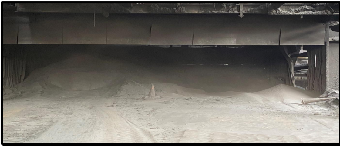
Figure 5 - Pug Mill Floor
