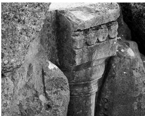
Fig. 11. Side view of the Lion Gate relief, showing curved saw cuts on the left side of the entablature and the Left Lion.
