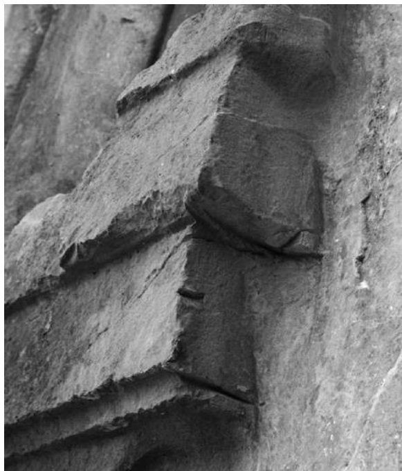
Fig. 13. Three short, curved saw cuts on the right side of the right altar.
