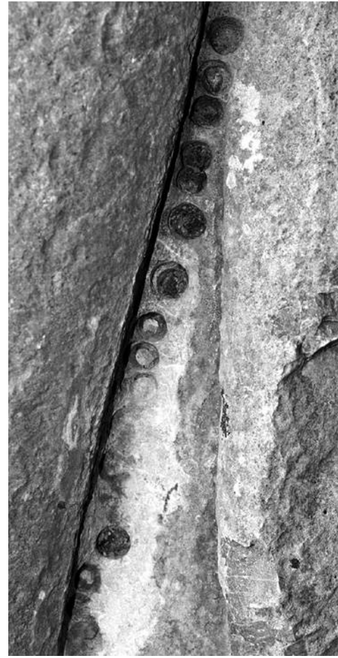
Fig. 16. Series of drill holes with unknown mortar-like filling between the hind leg and tail of the Right Lion.
