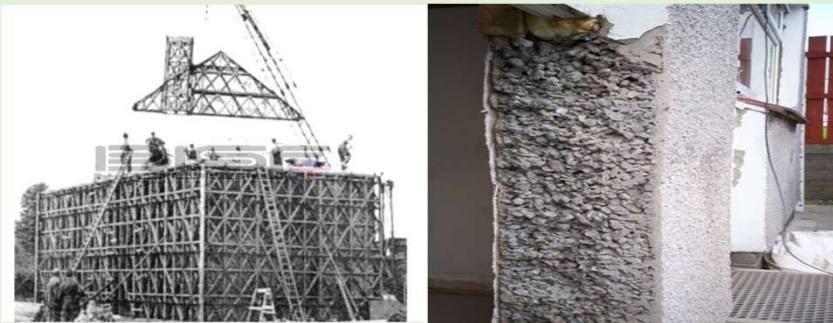
Fig. 1 Pre-fab shuttering Fig. 2 250mm External wall
