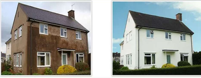
Fig. 7 External Wall Insulation before and after
