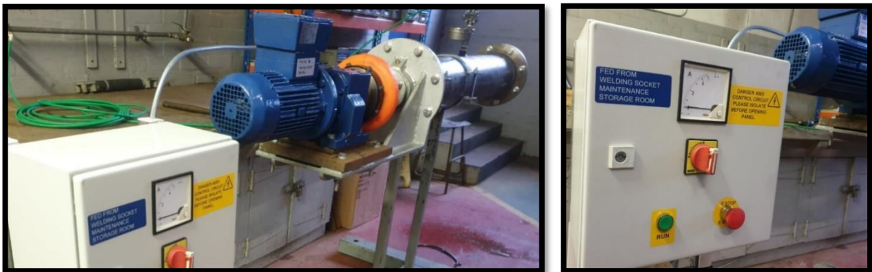
Figure 16 - Ammeter Added to the Motor Circuitry of Conveyor Test Rig
