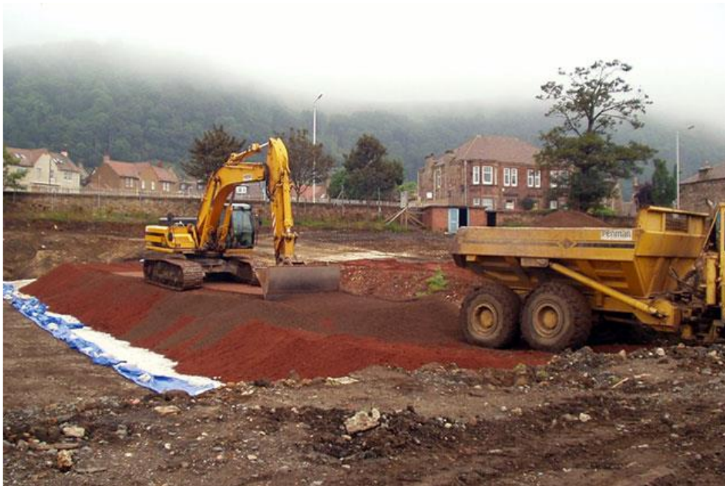
Image of a 'capping layer' (Soilutions Ltd, 2017a)
