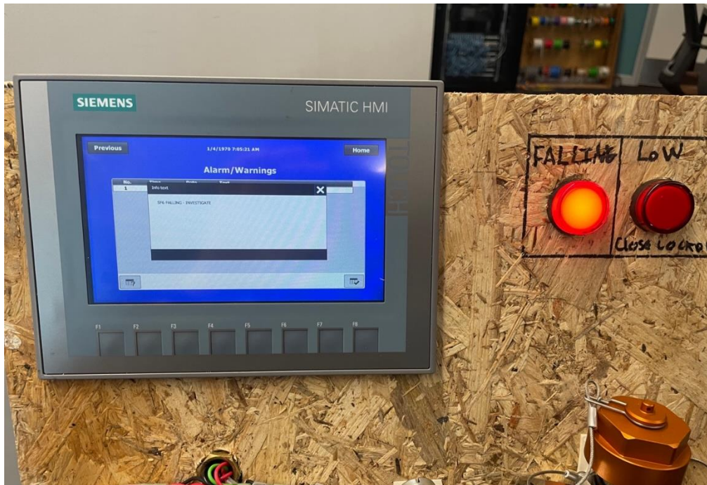
Figure 35: Warning notification Label/instruction
