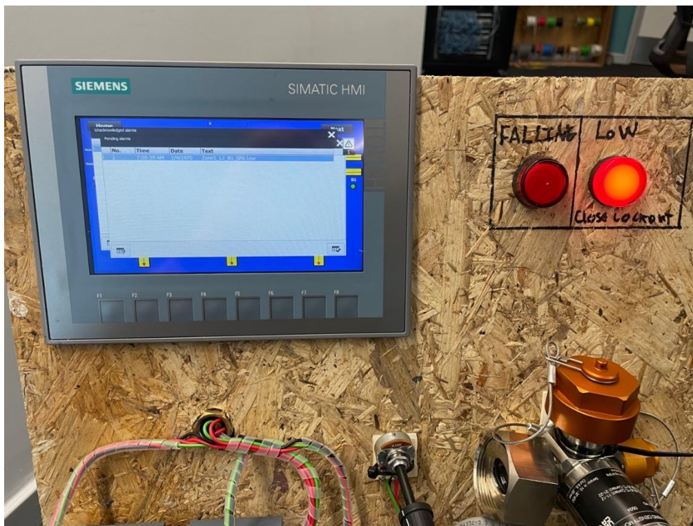
Figure 36: Immediate alarm pop up notification
