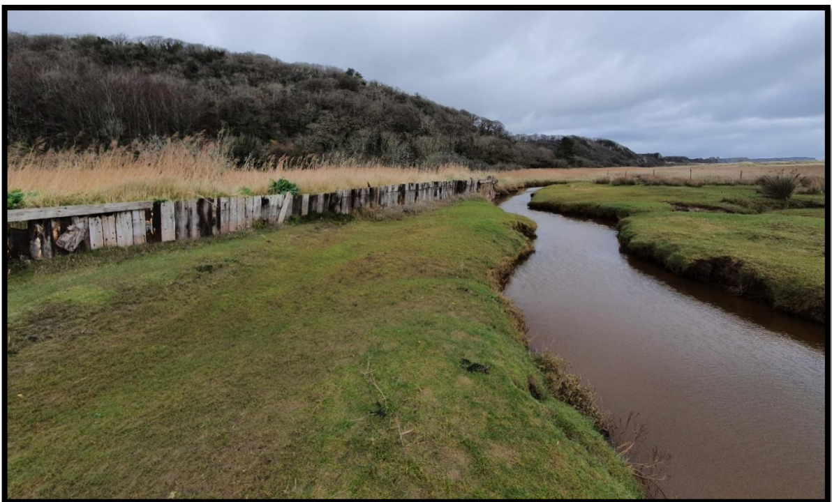
Figure 2.10 - Bund embankment between freshwater swamp and saltmarsh (Drummond, 2022)
