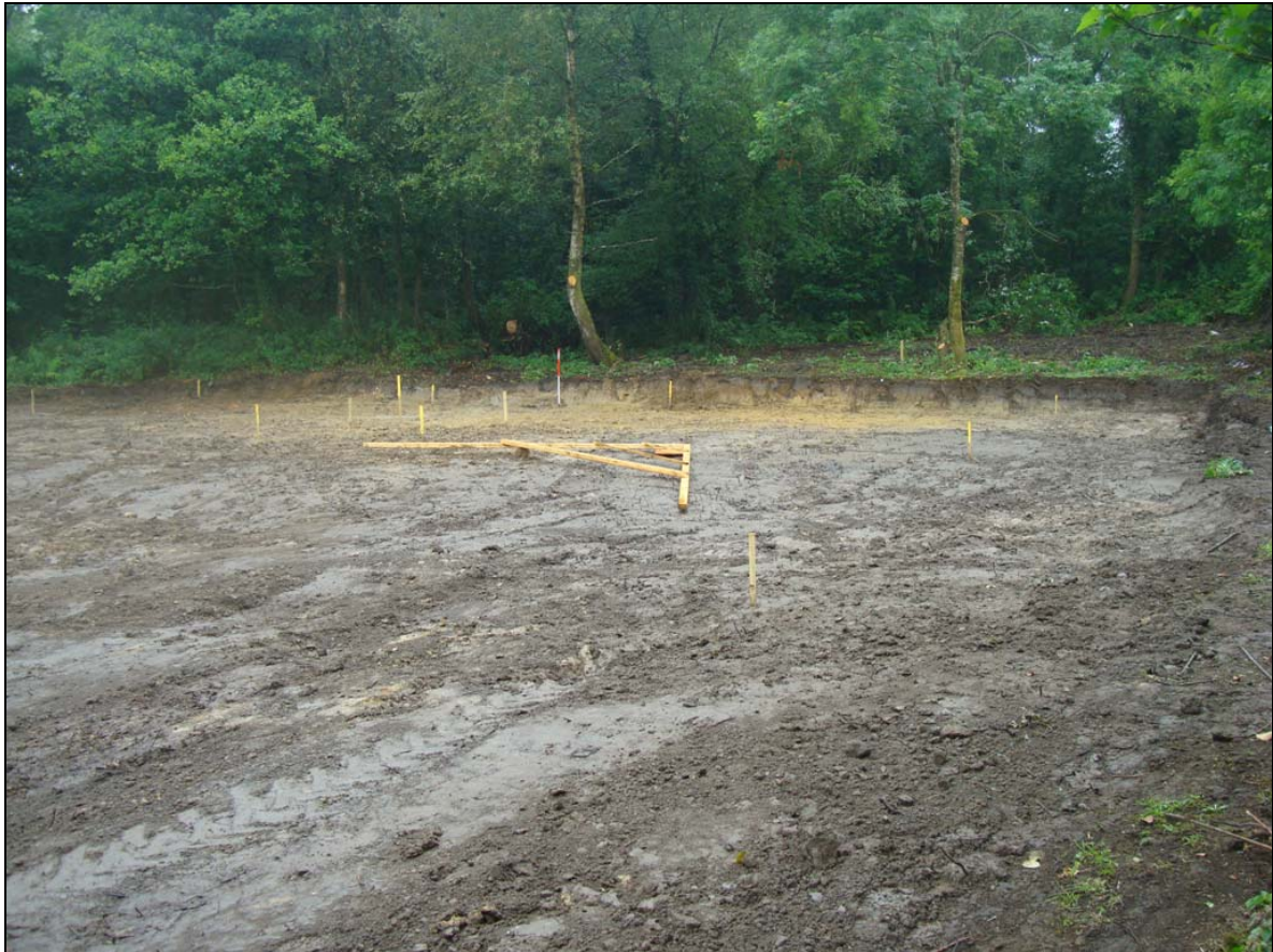
Plate 15: CYB15 – The western development area after levelling of ground, looking east
