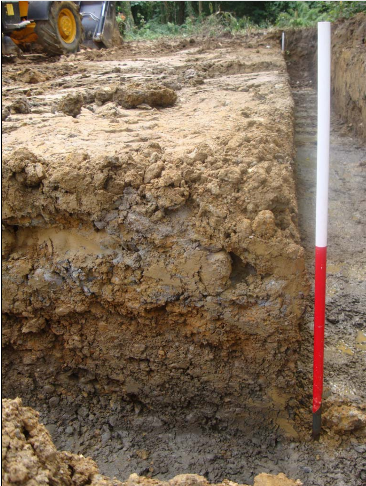
Plate 17: CYB17 – The western development area after levelling of ground, looking east
