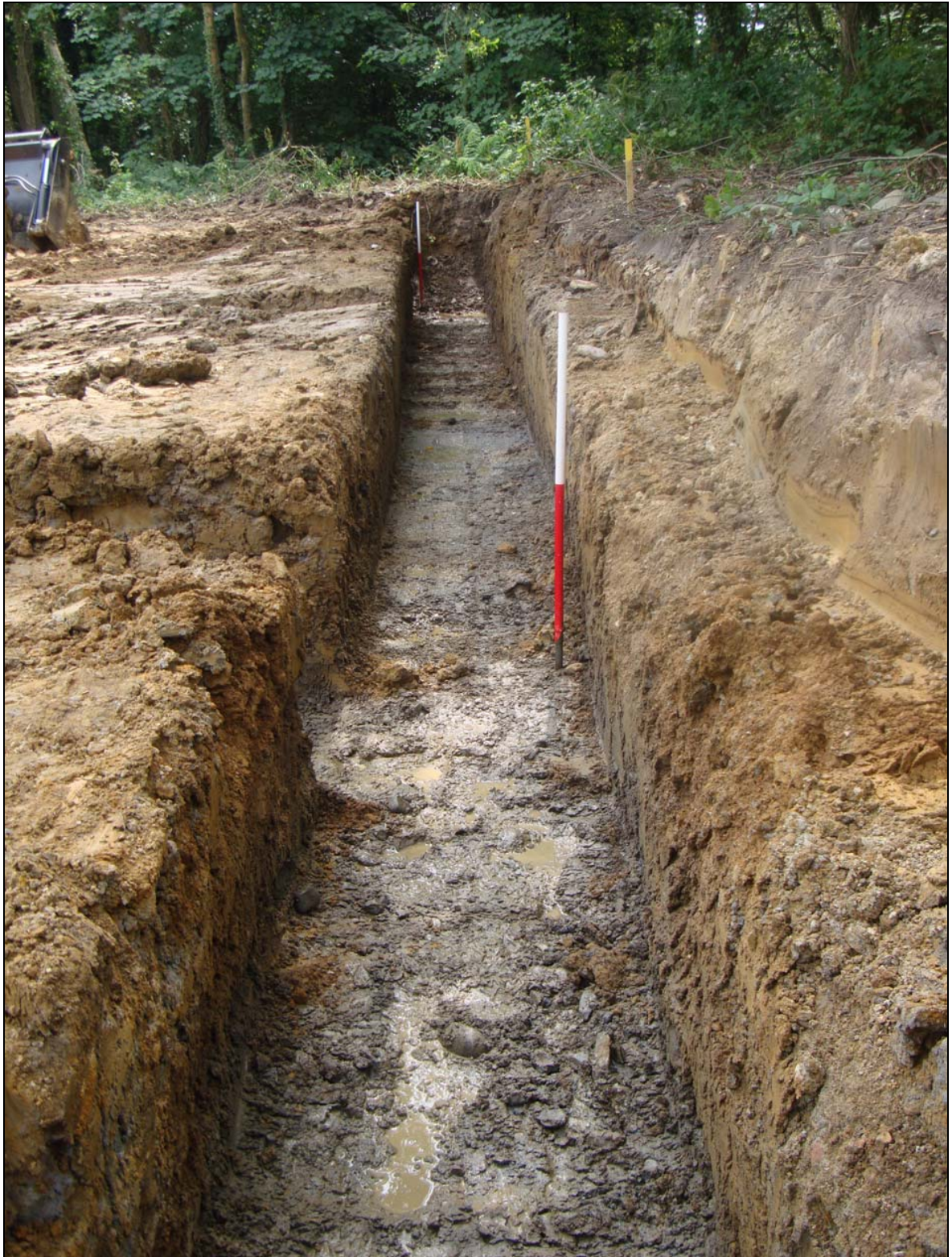
Plate 16: CYB16 – Footings for House 3, looking east
