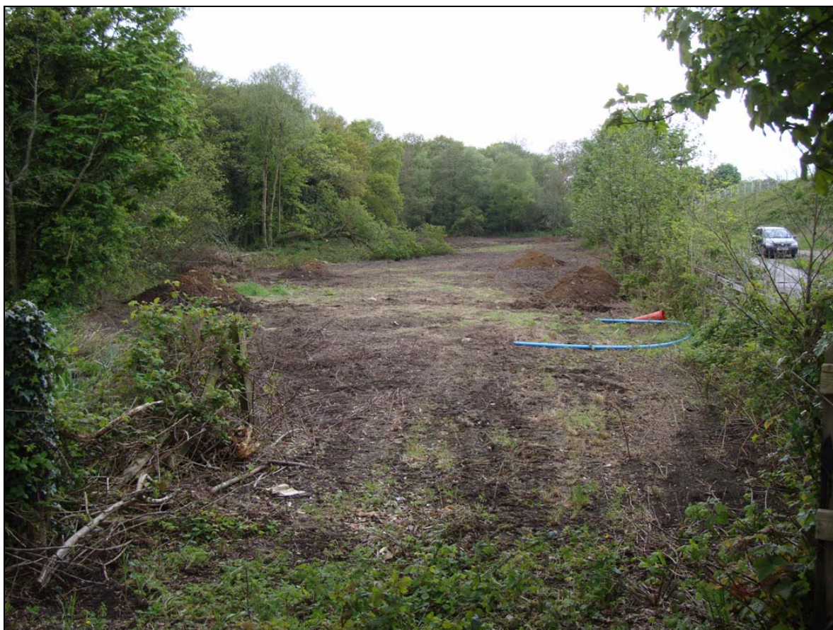
Plate 3: CYB03 – Development plot showing test pits looking west
