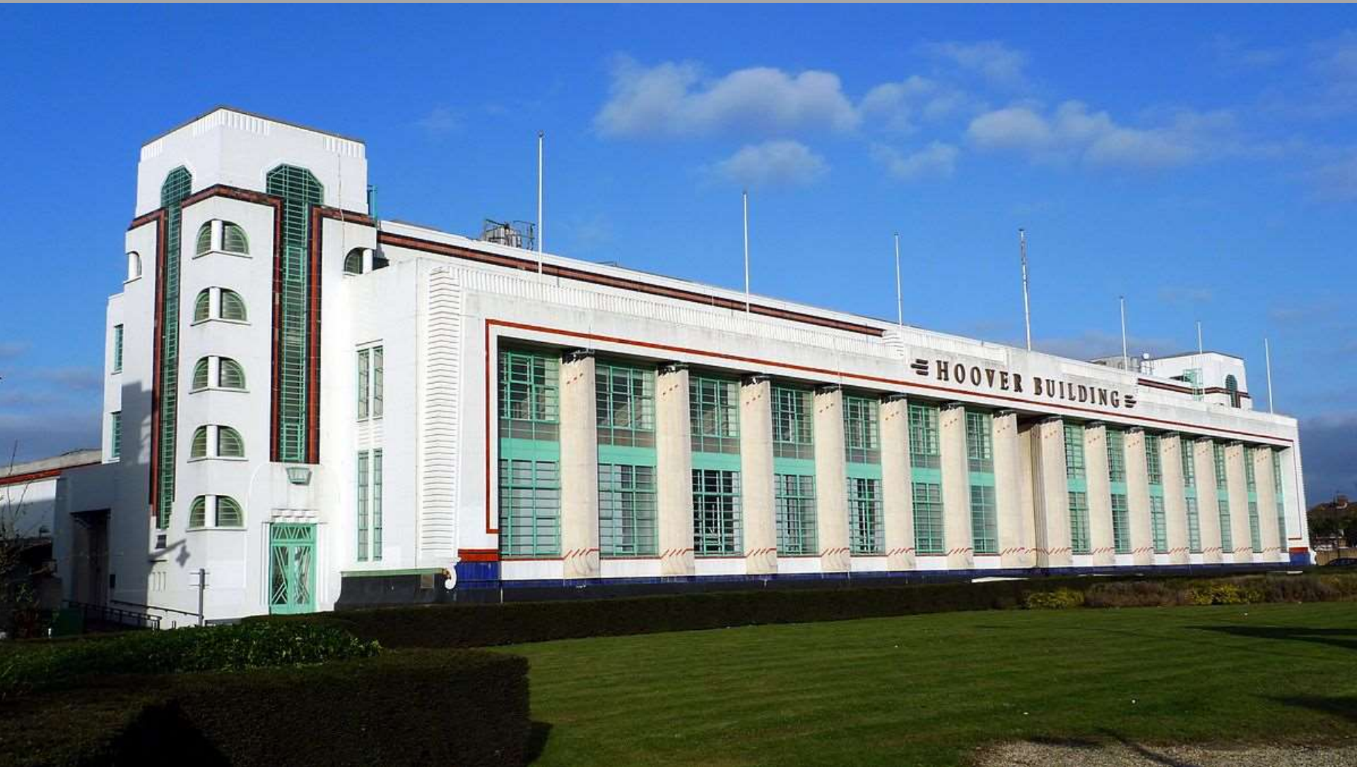
Wallis Gilbert and Partners, Hoover Factory, Perivale London, 1935
