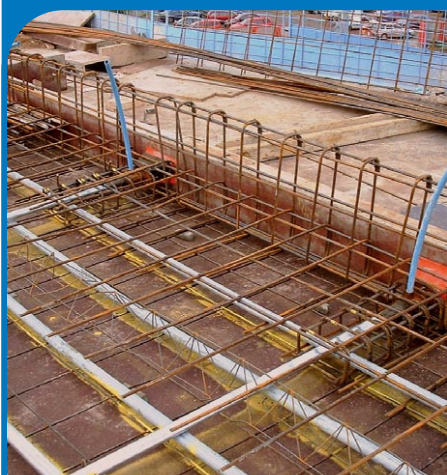
Bonded system before pouring concrete. Courtesy of Freyssinet.
