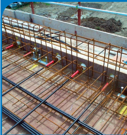
Unbonded system before pouring concrete. Courtesy of Balvac.
