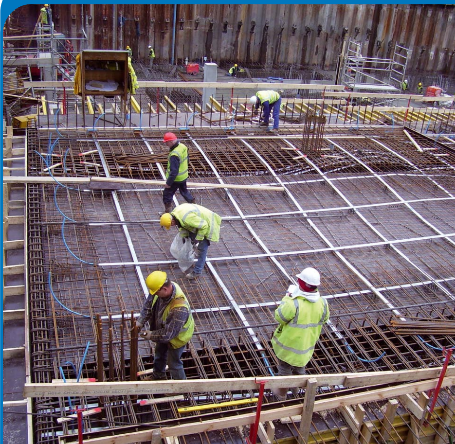
A typical PT beam and slab under construction. Courtesy of Freyssinet.
