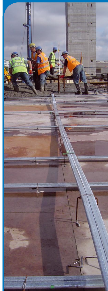
FIGURE 15: CONSTRUCTION JOINTS
