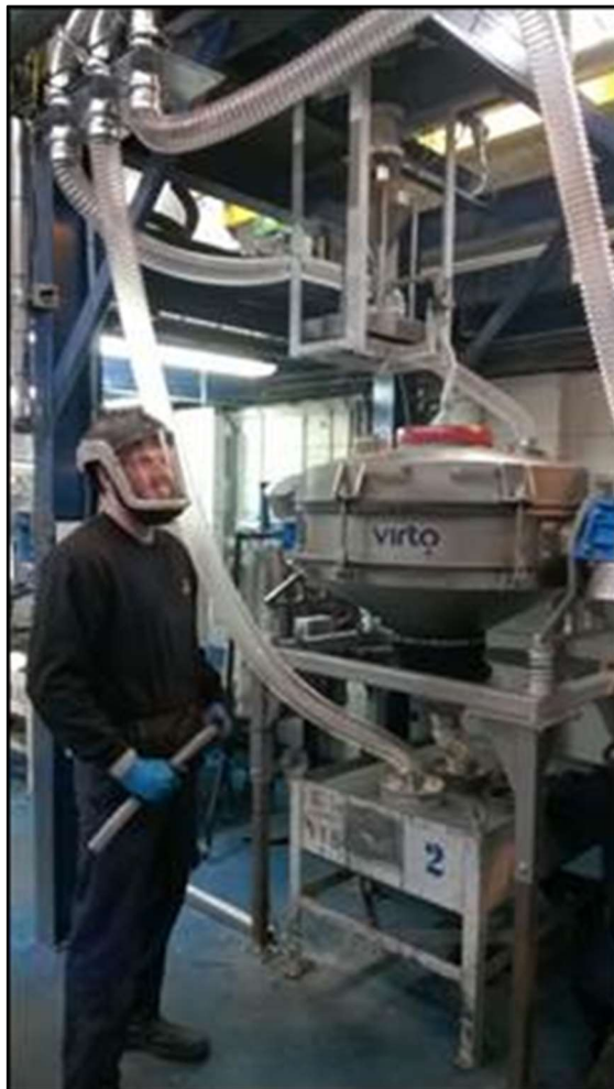
Figure 27 - Set up of Trial using Virto Screener At WCL
