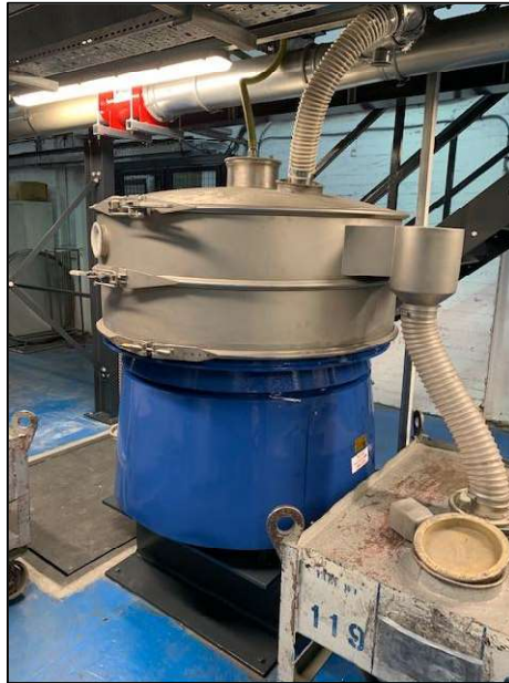
Figure 60 - Vibratory Screener Installed
