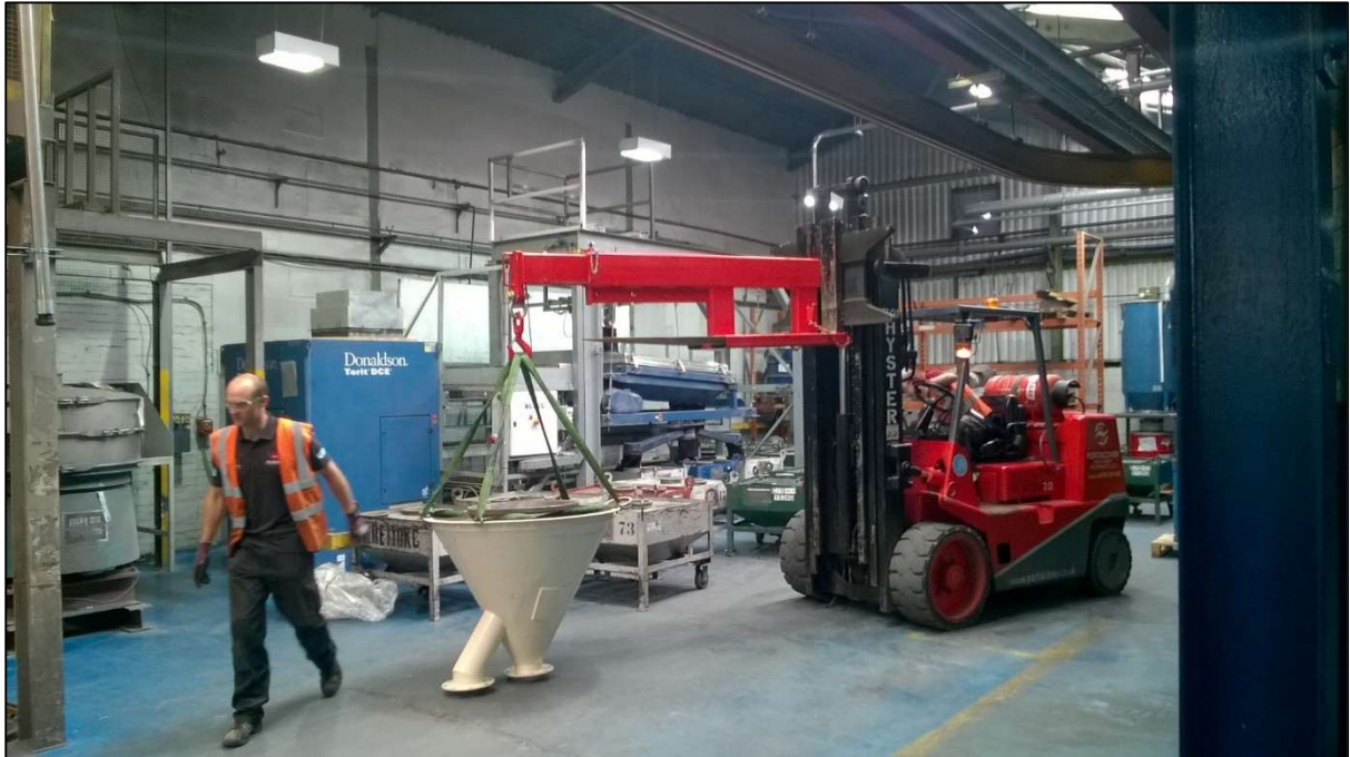
Figure 58 - Forklift Installation of Air Classifier Base
