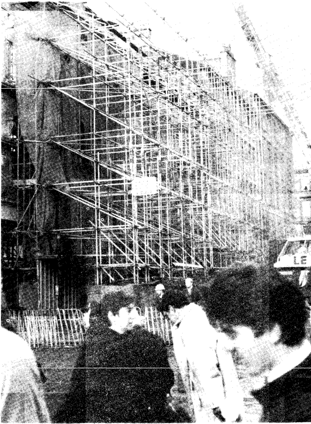
Figure 2 Scaffold tube and coupler system. The general public is excluded and the base of the shore is protected.
