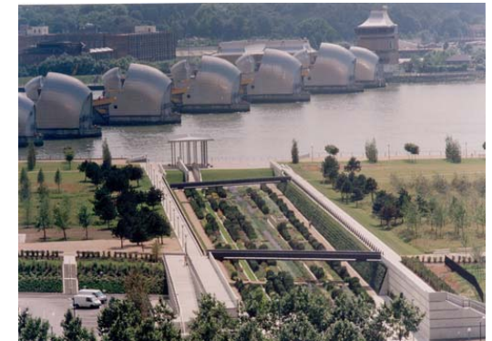
thames barrier park – linear landscaped space
