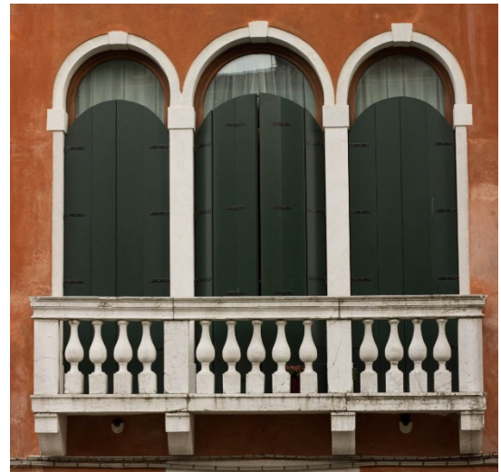
Fig4: Balcony with balusters
