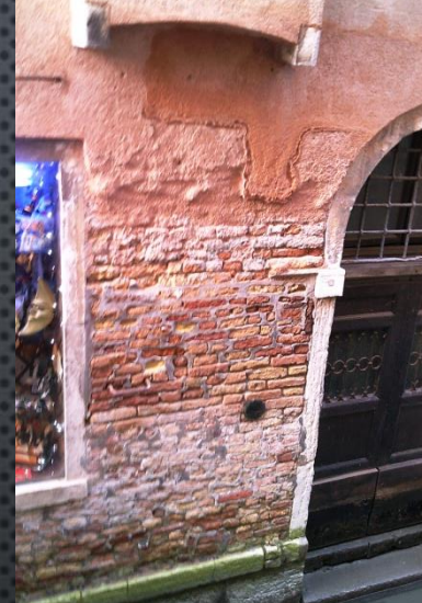
IMAGES OF VENICE ABOVE MIGHT BE EXTREME, BUT THE OTHERS OF SOUTH WALES ARE EVIDENCE THAT RISING DAMP IS NOT THE MYTH THAT IS BEING ARGUED.
