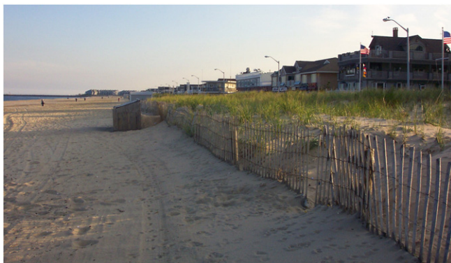
Fig. 1. Common initial sand fence deployment for dune building purposes, New Jersey.
