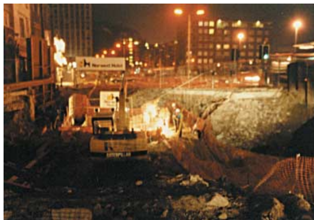
Figure 1. October 1992: deep excavation by floodlight in the midst of Dover's major road-works. (V. Fenwick)
