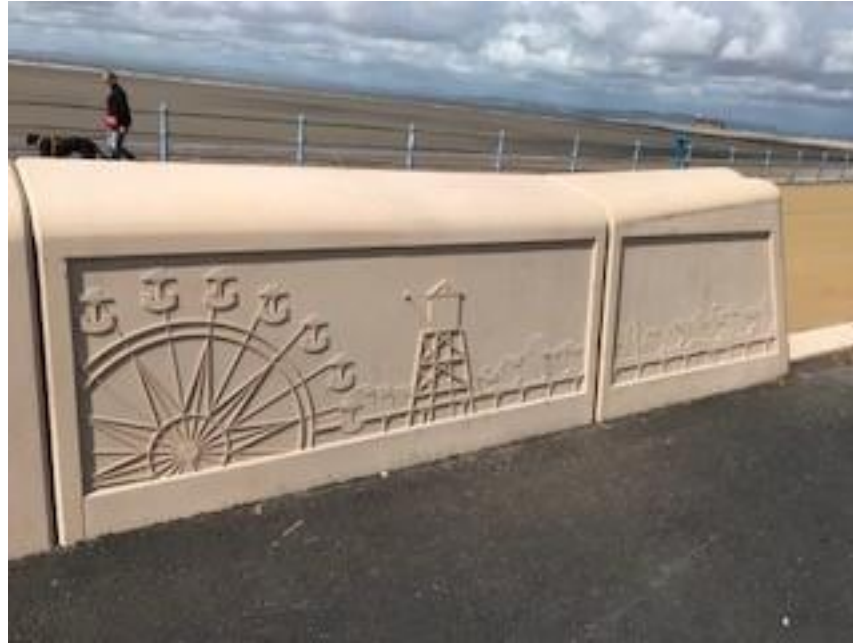
Examples of Reckli patterns on the rear of wave return walls
