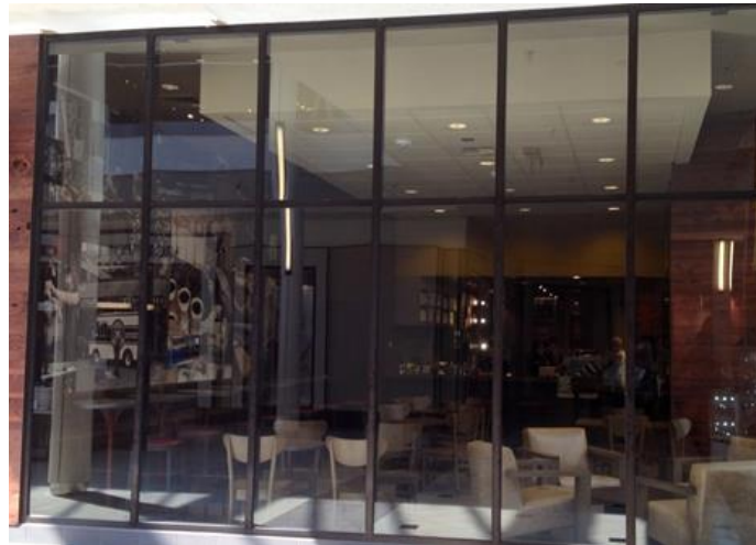
Curtain wall storefront (Advanced Glass Expert, 2016).
