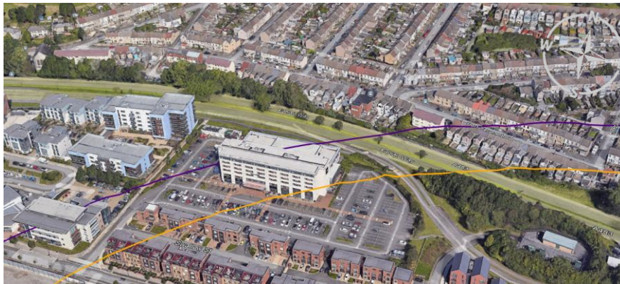
Figure 5 - Circular QD boundary intersecting the hotel.
