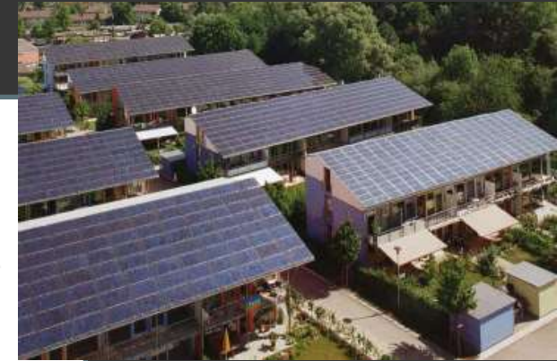
Architects Rolf Disch, Housing Freiburg Germany
