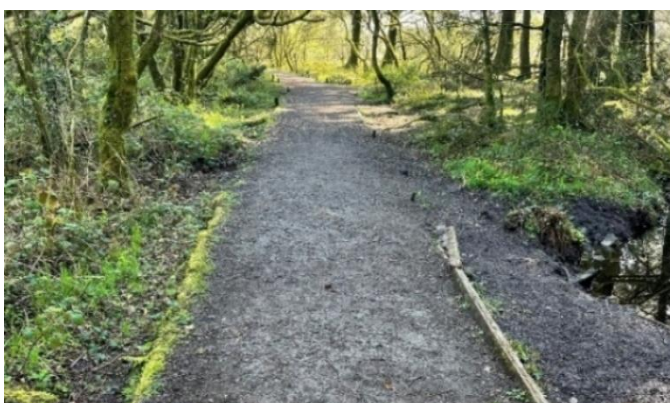
Figure 25 Path next to stream damage (Egan, 2023)
