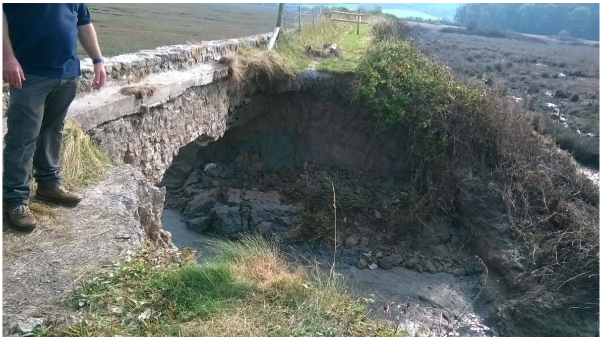
View of breach in sea wall/defence
