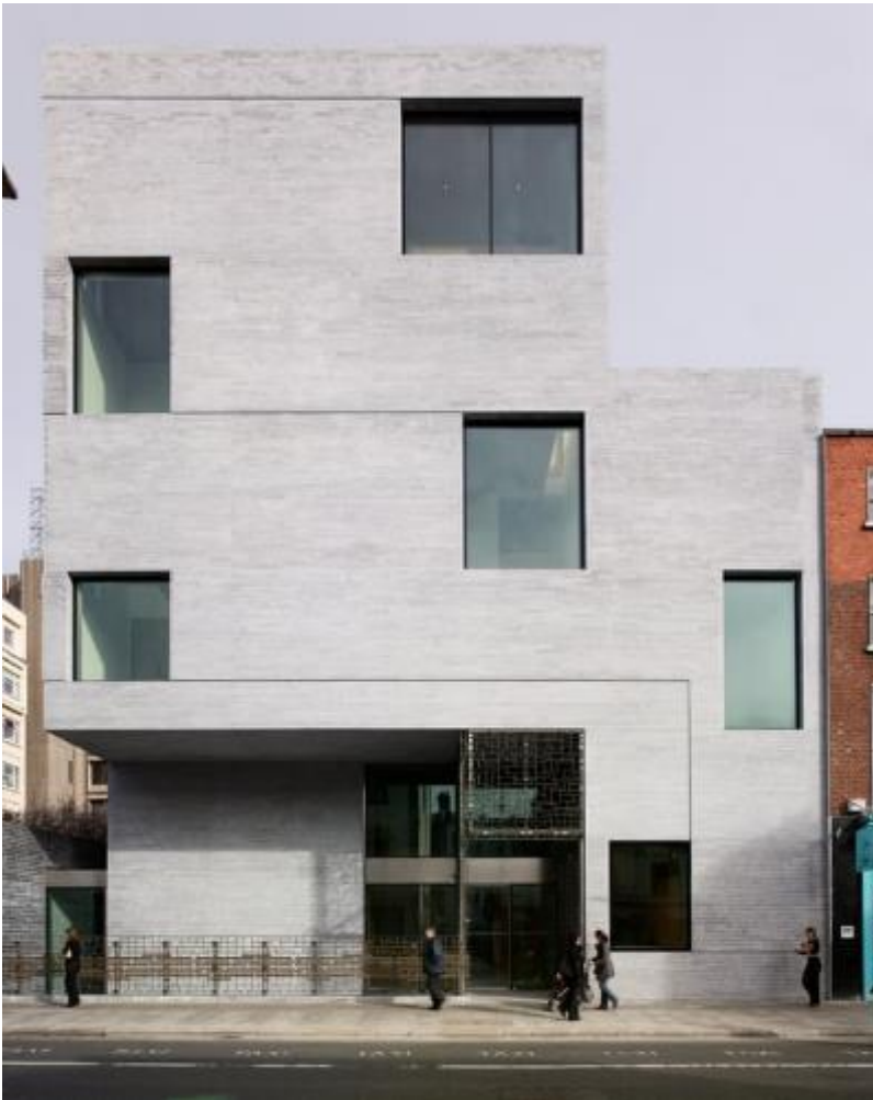
Department of Finance in Dublin by Grafton Architects, 2009
