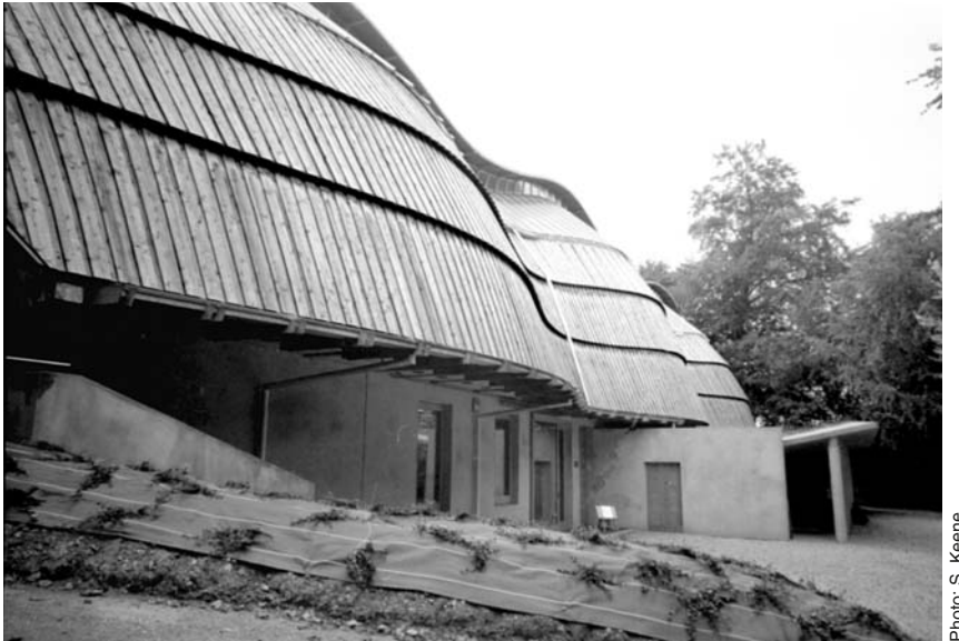
Fig. 1.3 The Downland Gridshell (2002). An award winning building made of a grid of oak laths, it houses the collection, conservation, and teaching activities of the Weald & Downland Open Air Museum
