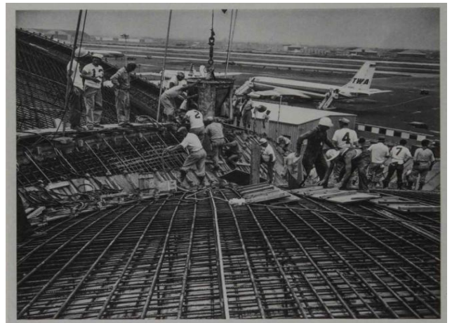
Figure 2: Concrete shell creation. (Ringli, 2015, p. 102)
