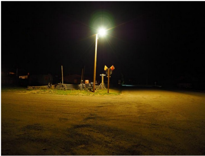
Figure 16: Evluma Areamax 40 Watt, LED, shielded, 3000 Kelvin, 3500 lumens, in Stanley, Idaho. Installed in 2015. Photo: Mayor of Stanley.
