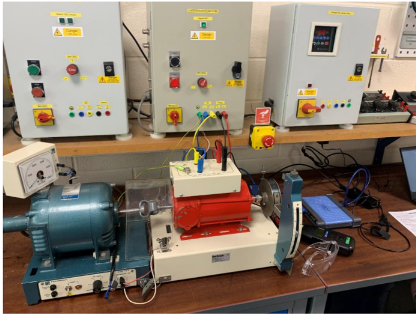
Figure 2: Practical set-up of DC motor supplied by a Parker 512c drive
