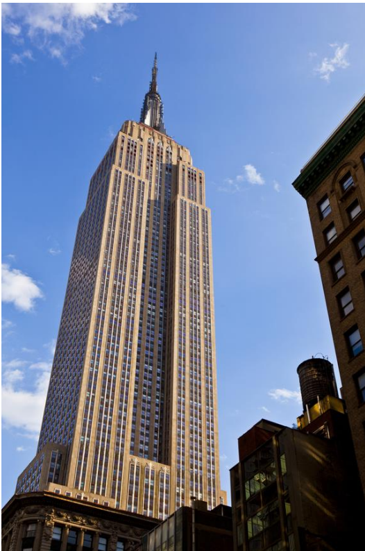
Figure 1 – The Empire State Building (Alltickets.com, nd)
