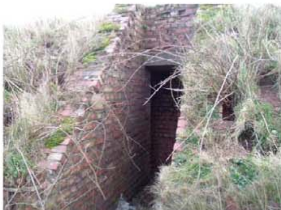
Plate 3 WW2 structure that may support roosting bats.
