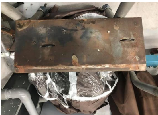
Figure 3-20 Control Board from Source
