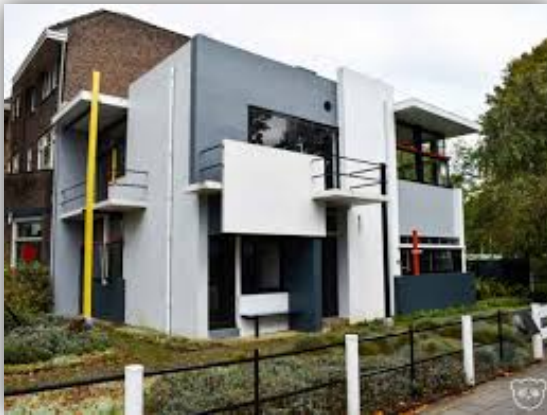
Elevation of the Schroder House showing the floating panels and coloured lintels- (Gerrit Rietveld's Schröder House: Perfect Harmony in a Home | The Art Minute, n.d.)
