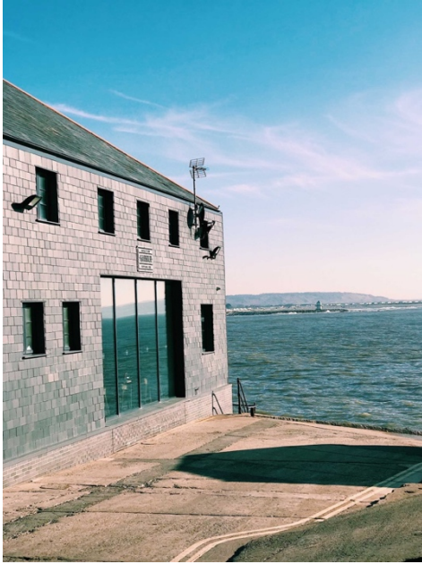
Figure 46: The Jennings Warehouse
