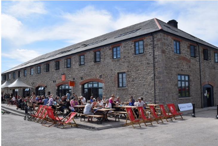
Figure 44: Jennings building Porthcawl
