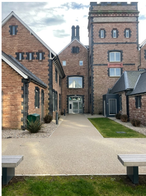
Figure 49: The Links restored listed wing
