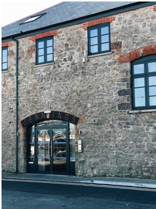
Figure 41: The Jennings Warehouse
