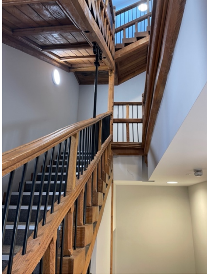
Figure 25: The Links reconstructed original staircase
