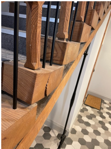
Figure 28: The Links worn original timber
