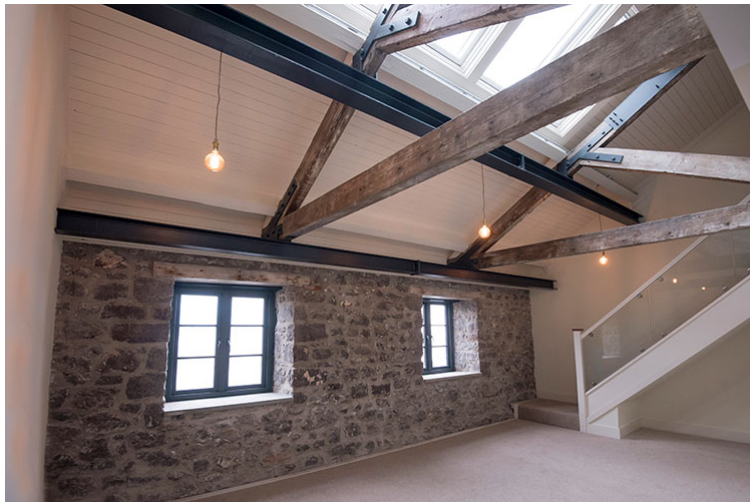
Figure 47: Jennings building Porthcawl
