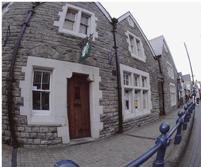
Figure 34: Old Police Station Porthcawl
