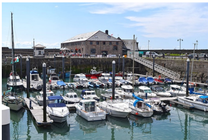
Figure 42: Jennings Warehouse Porthcawl
