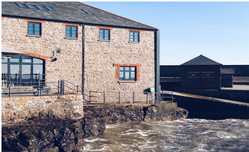
Figure 43: The Jennings Warehouse
