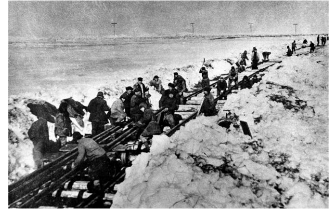
Prisoners building a section of the railway during winter. (1900/1910s), History of Russia: How the Trans-Siberian Railroad Reshaped the World
