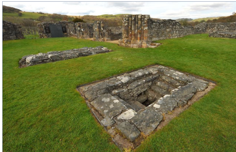
Fig. 33: The holy well at the crossing of the abbey church, looking north-east. It has two flights of steps down to a square cistern in the base with the openings of two stone-lined conduits, one from the south bringing the water in and one to north for the out-flow. The eastern set of steps leads from the high altar (to the right), while the other to the nave. This suggests that the holy well was intended to be part of a ceremony with monks officiating.
