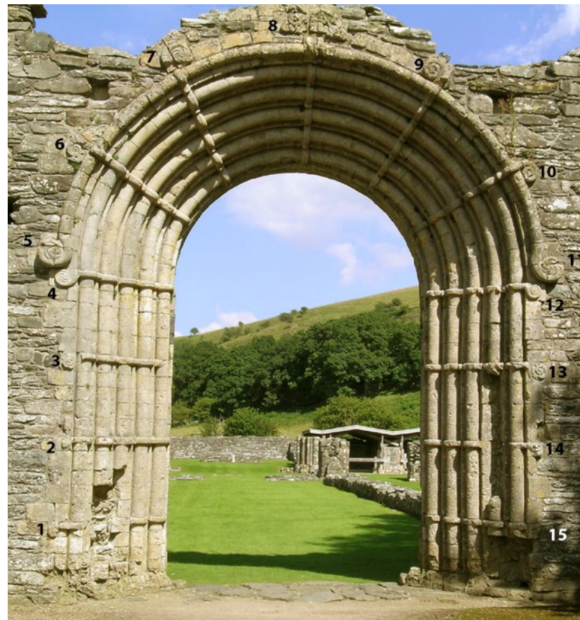
Fig. 40: The western portal of the abbey church executed in Dundry stone. It is stylistically Transitional between Early Gothic and Romanesque.
