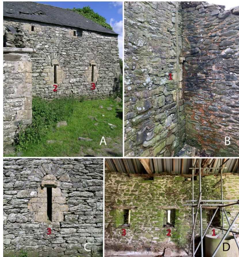
Fig. 69: Photographs showing details of the medieval walls and ventilation. They were made from Dundry stones taken from ruined abbey buildings.
