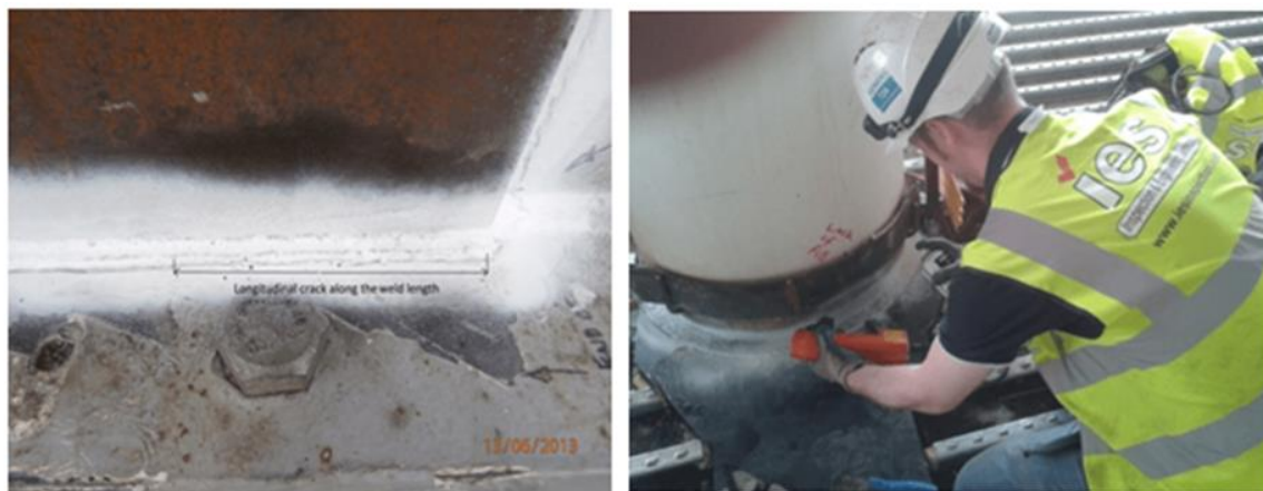
Figure 17 -MPI pipe testing and crack detection (TWI Global, 2019)
