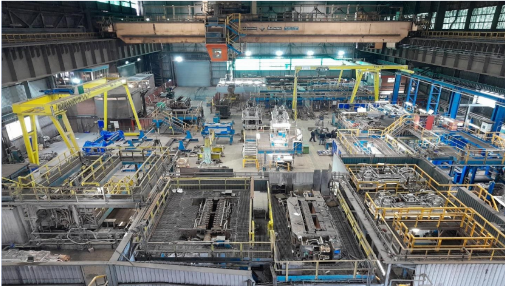
Figure 6 Process Bay Workshop
