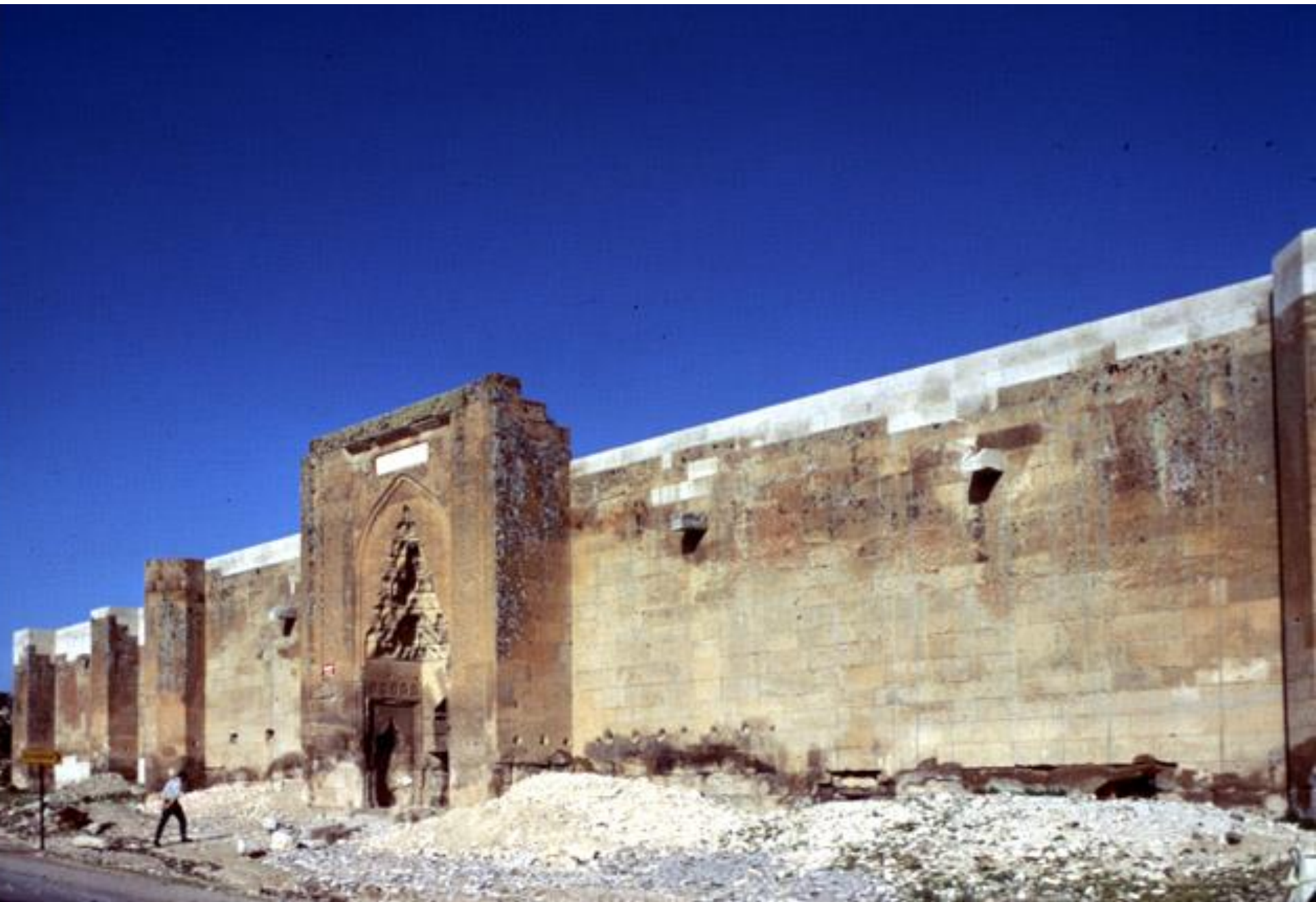
Agizkara Han, near Aksaray Façade and portal
