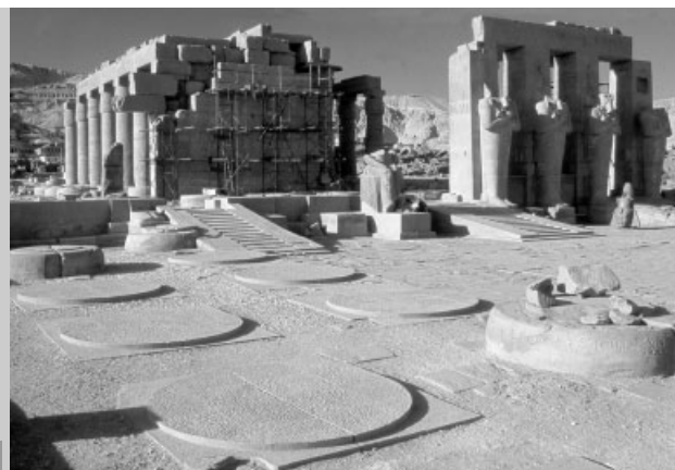
28. Restitution of the bases of Ramesseum's columns, an example of reversibility in restoration, facilitating a better legibility of the ancient temple's architecture.
