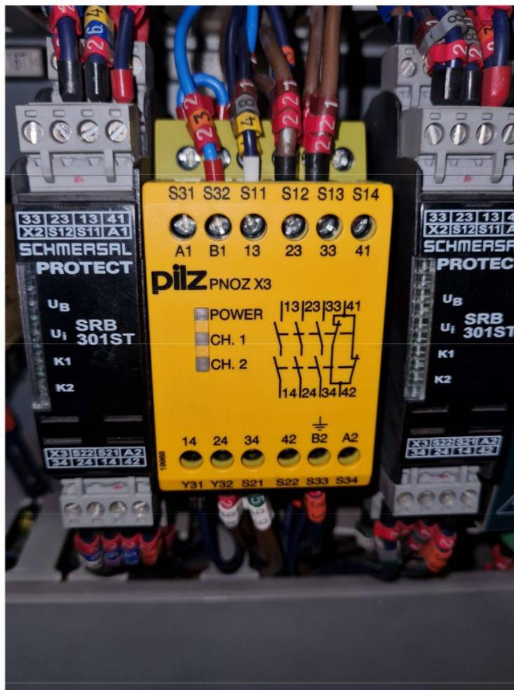
Figure 17 - PILZ PNOZ X3 Safety Relay
