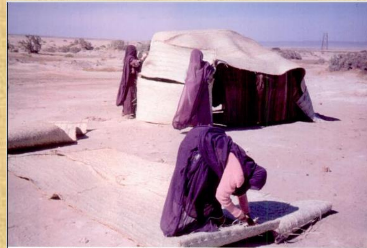
Pl. 11.1: Building the 'Ababda abode: adding mats to the wooden frame.
