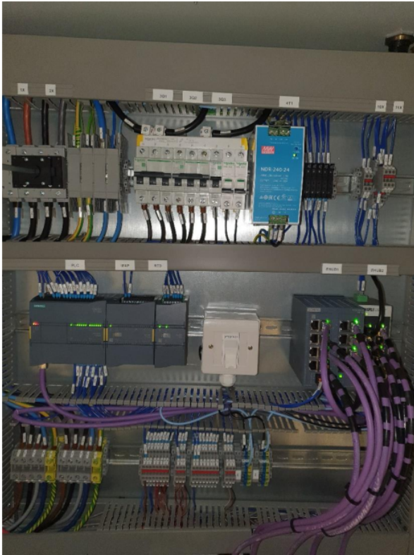
Figure 13: Main Panel Hardware Install
